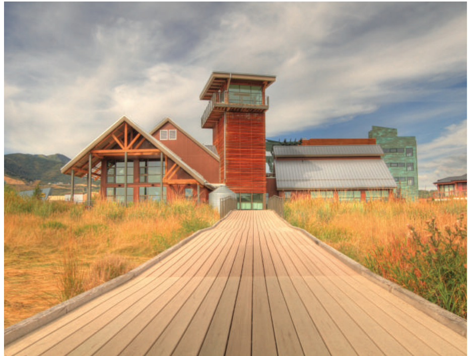
The 10,000-square-foot, LEED Platinum education center at the Swaner Preserve and EcoCenter in Park City, Utah is a key attraction of the 1,200-acre wetland ecosystem nature preserve. Photo courtesy Swaner Preserve and EcoCenter
